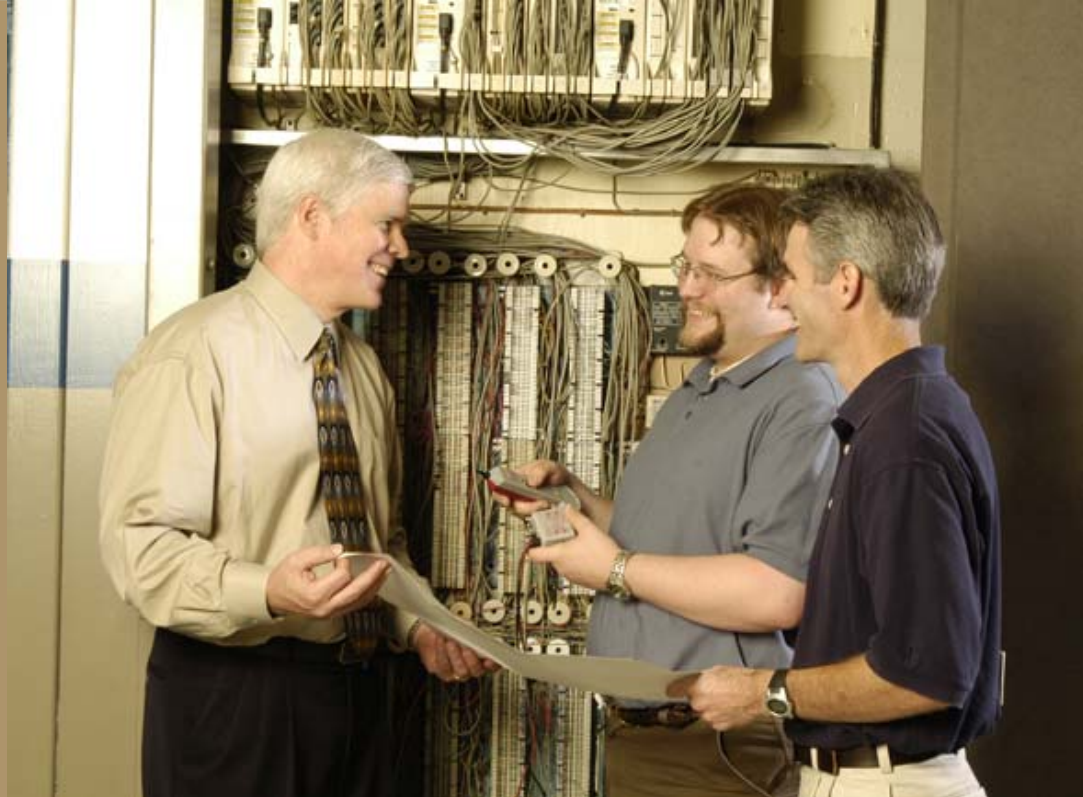
Aircom Manufacturing, Indianapolis
