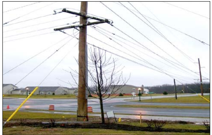
Do not plant trees near overhead utility lines unless approved by a utility forester. This will help eliminate the need for harsh pruning measures as the tree matures.
