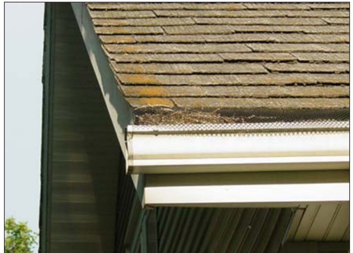
Figure 3. Wildlife can damage houses and other structures. Nuisance wildlife control operators usually either repair the damage themselves or subcontract that work to another business.
