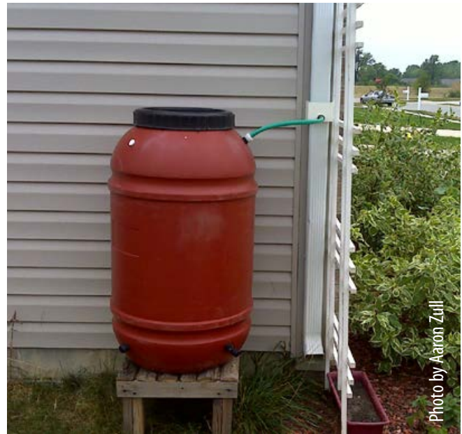
Figure 15. Homeowners can use rain barrels to collect rainwater. This helps reduce surface runoff after rain events and allows homeowners to store water for use around their homes. This saves water and money by avoiding using water from the tap.
