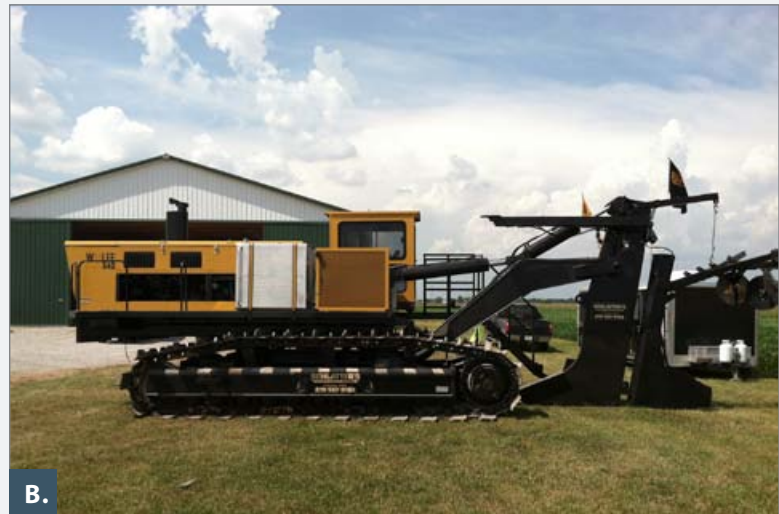
Figure 3.14. A. This photo shows tile drainage being installed. The perforated yellow tube is installed underground, almost level, but with a slight slope so it drains to an outlet. It is deeper under swells than under depressions. The placement of the tube in the soil is guided by laser beam or enhanced GPS (RTK) technology. B. This image shows a larger machine with the working parts out of the ground. The machine moves toward the left. 3.14A provided by Tom Bechman; 3.14B provided by Joey Schlatter.
