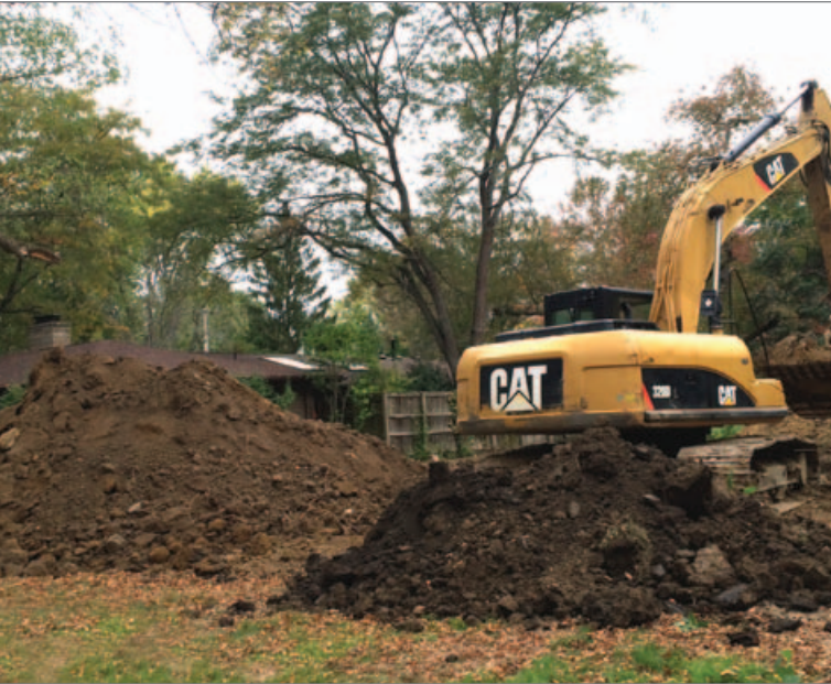
Figure 4.1. On this construction site an excavator has stockpiled A horizon material (front of excavator) and A and B horizon material (left of excavator).
