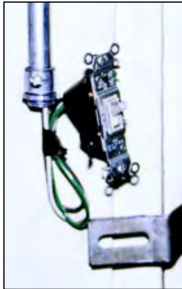
Electrical wiring protruding from its conduit and taped to “hang” instead of being installed properly
