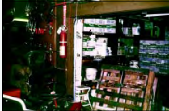
Example of cluttered path to fire extinguisher
