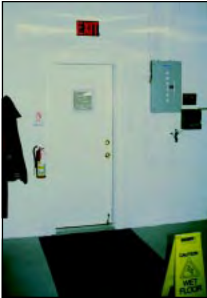
Make sure all exits are marked clearly and that the path is clear
