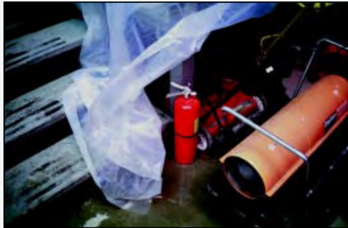
Fire extinguisher sitting in water on the floor
