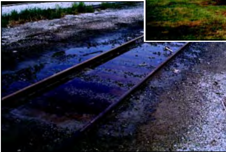
Spill resulting from irresponsible transfer of chemicals
