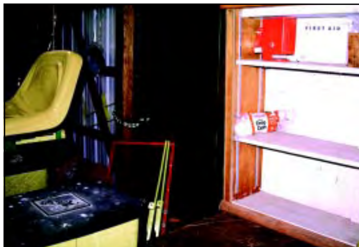
Unacceptable: Path to exit is cluttered and door is padlocked
