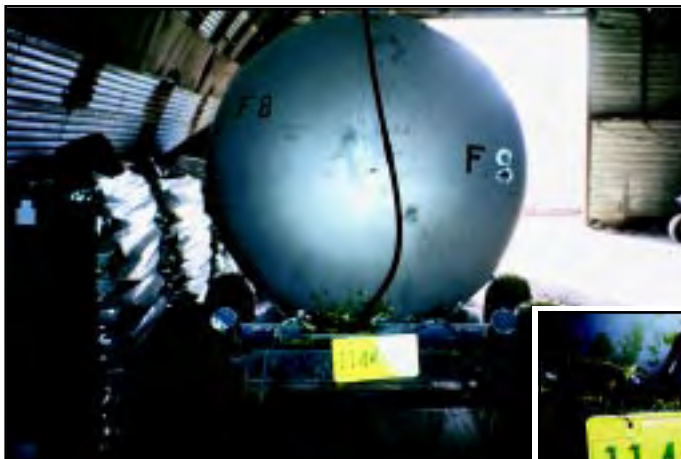
Chemical ate through hose (inset) and flowed out the back of the building into a tile leading to the city pond (see adjacent page).
