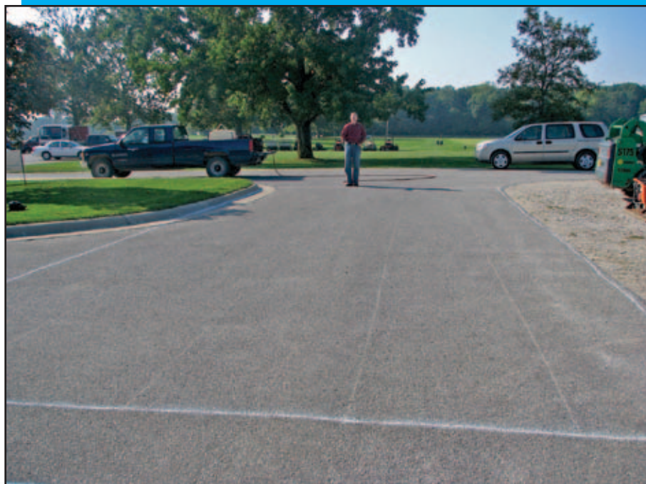
Using pavement for your practice runs allows you to easily detect bad application techniques, which can be corrected.
