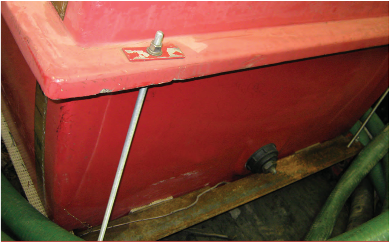
These metal rods link the fiberglass tank to the metal frame.
