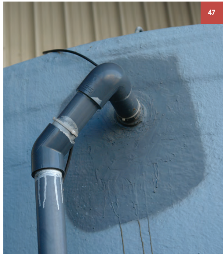
(Left) A sloppy tank repair job. (Right) This tank was properly ground, repaired, and repainted.
