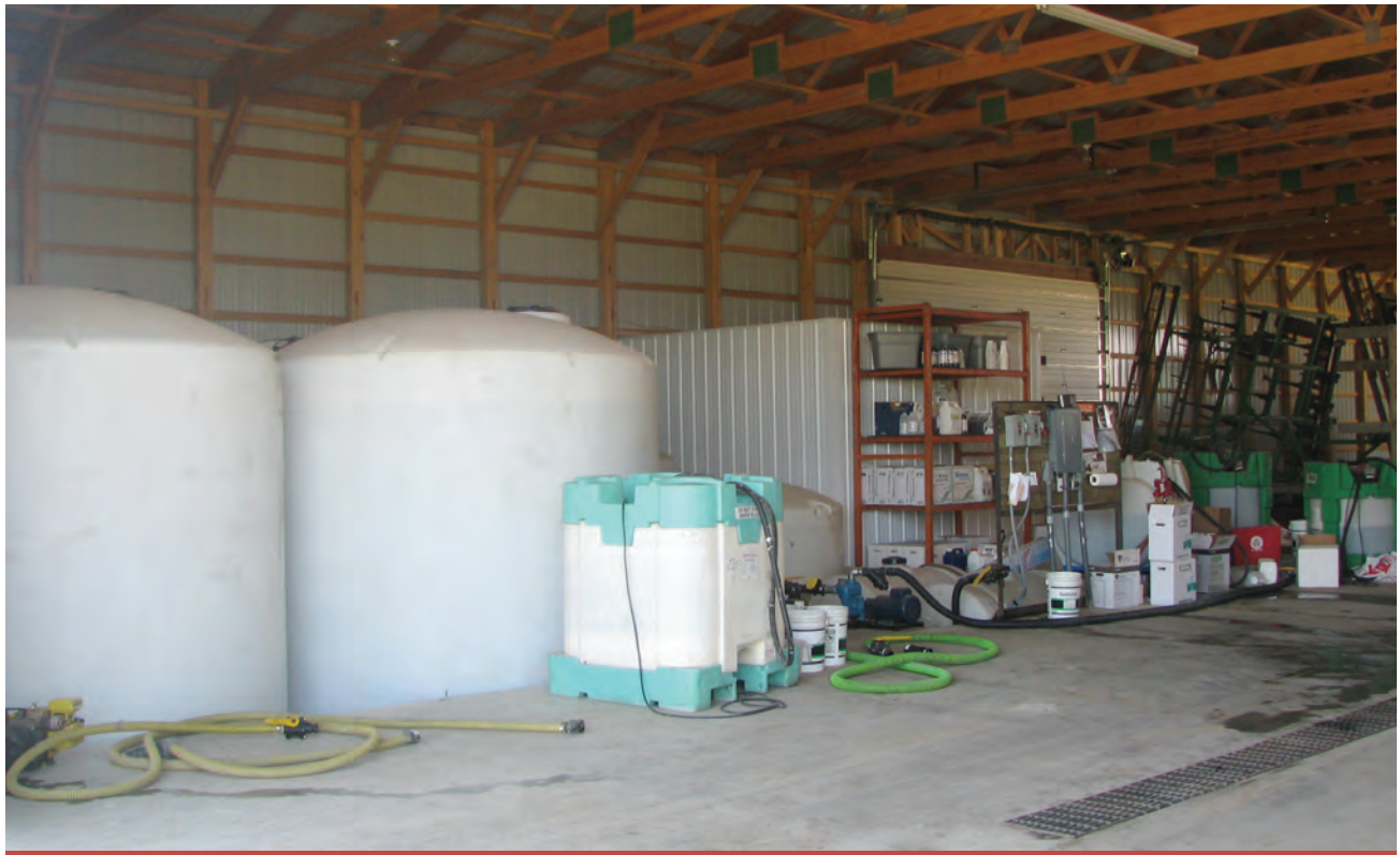
The large white storage tanks (left) are contained in a concrete pit that goes below ground level.
