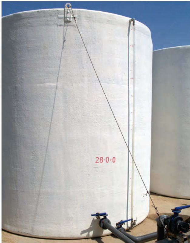
Tie-downs can secure tanks in the event of flooding or high winds.
