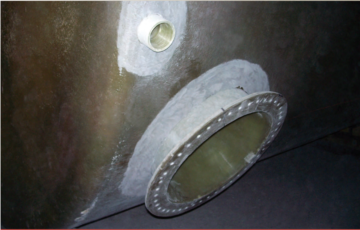
The fitting and manway are in place and ready to be glassed in on this tank. The white areas around each opening are where grinding was done to help the fiberglass and resin adhere, or bond, to the tank.
