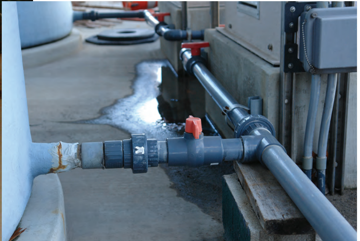
(Left) Make sure to support plumbing to limit pressure on tank fittings. A crack that's been repaired with putty is only a temporary fix.
