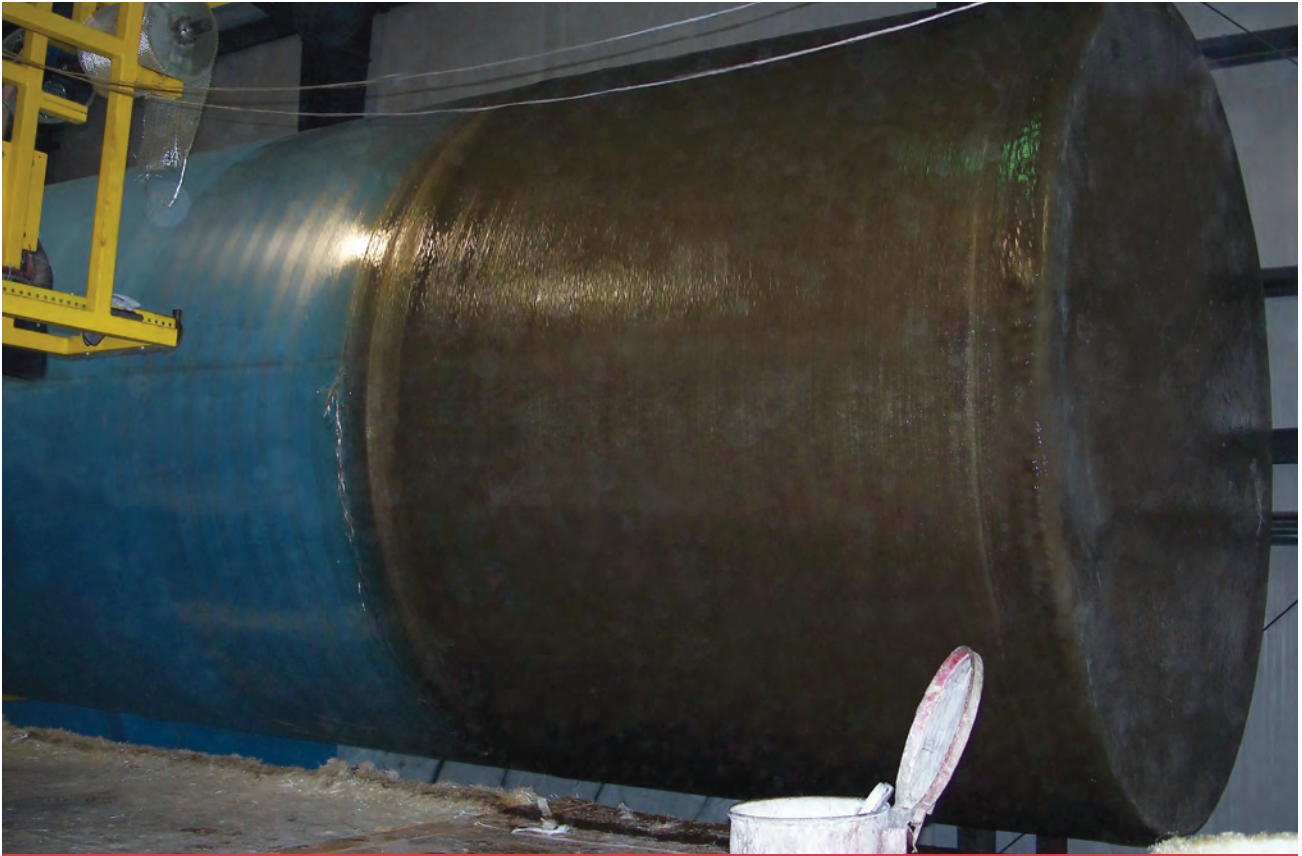
This tank has been wrapped with a woven mat and has had a hoop line added. It is now ready to be removed from the blue mold.
