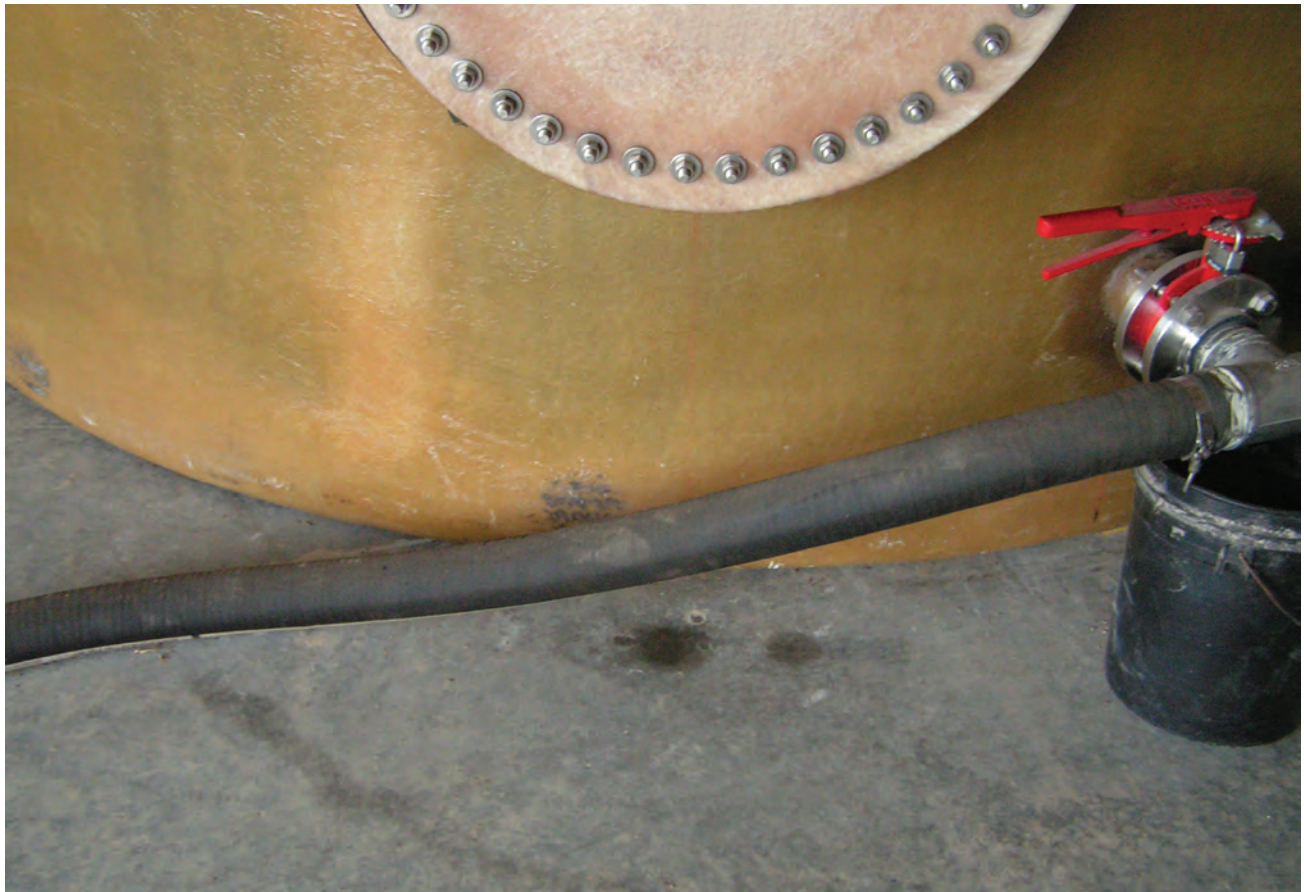
A small leak from this tank's manway allows the contents to accumulate on the concrete.
