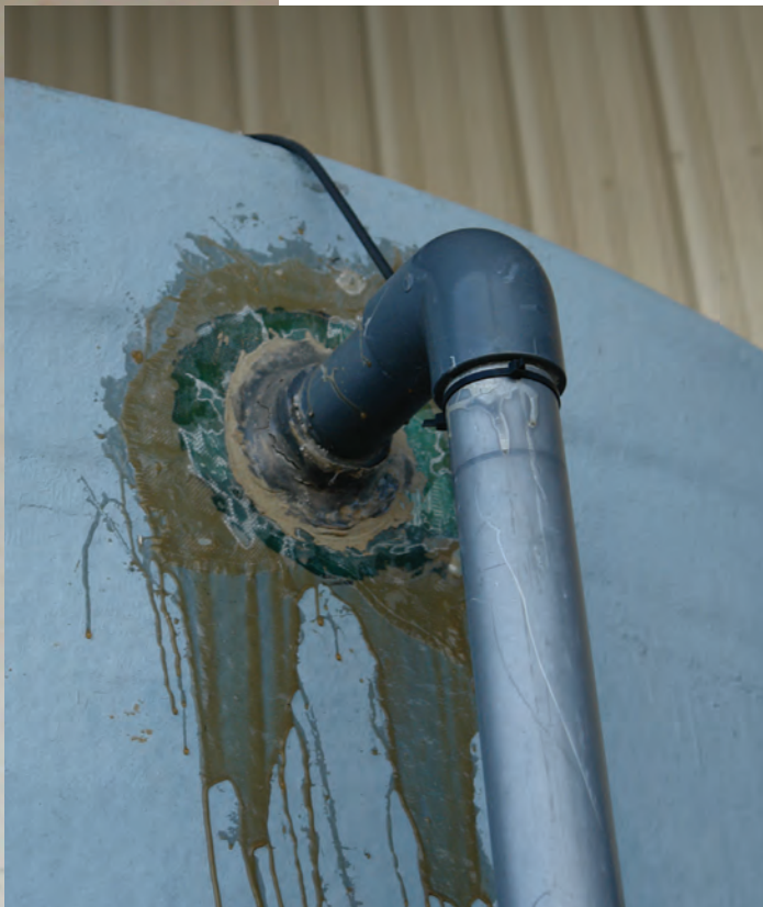
(Left) A sloppy tank repair job. (Right) This tank was properly ground, repaired, and repainted.
