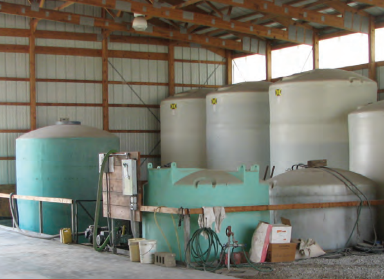
Poly tanks (left) and fiberglass tanks (right) each have advantages and disadvantages. Weighing the pros and cons of each are an important step in the selection process.
