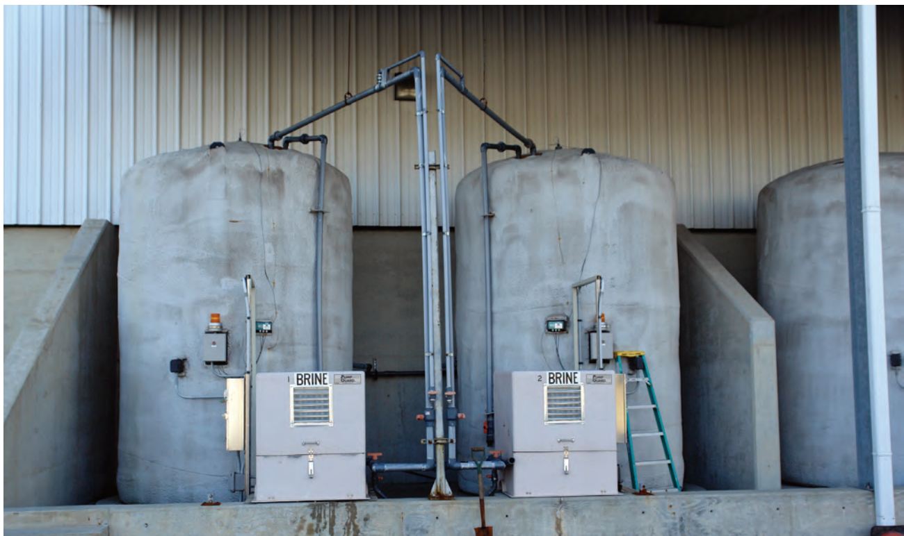
These brine tanks have been coated with insulation to protect their contents from cold weather.
