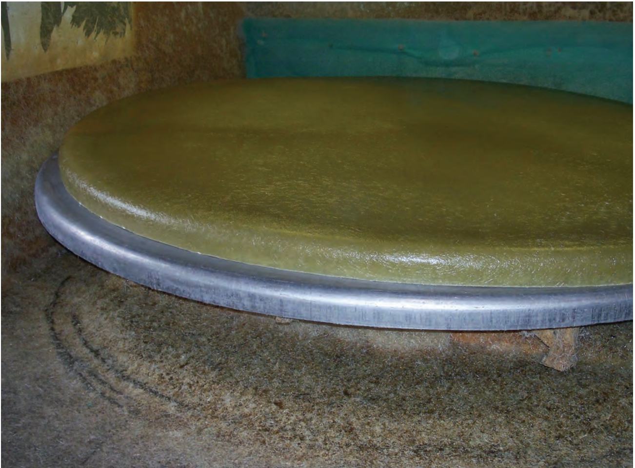
This tank bottom has just been popped off its mold.
