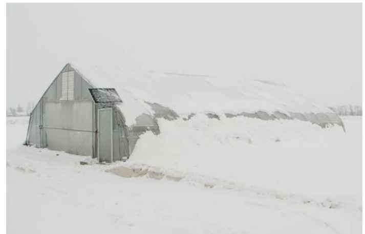
Figure 11. For this structure, snow blocks much of the south sidewall where light would enter, and is also shading the roof. A snow pile on the north side of the structure would provide insulation and not block so much light. (Photo by E. Maynard)
