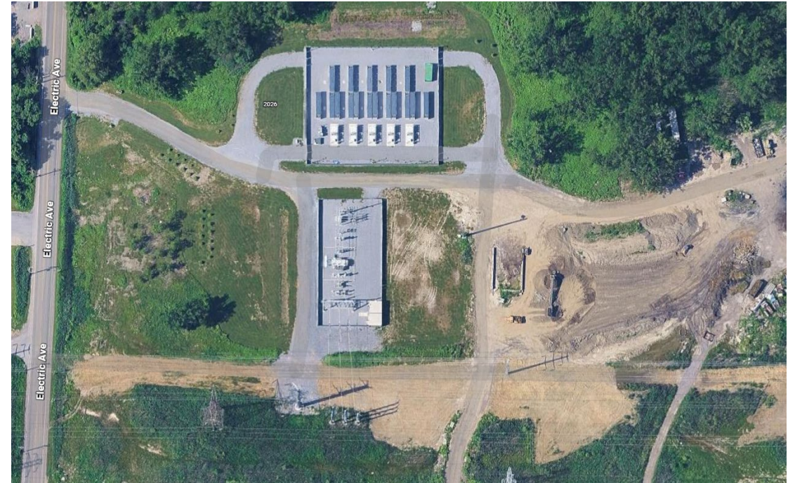
20 MW/45.6MWh LFP BESS in Erie County, NY (2023)
