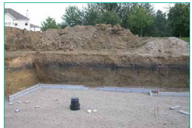
Figure 3. On construction sites, less productive subsoil (the upper and lower light-colored layers) is often brought to the surface and buries the nutrient-rich topsoil (the darker layer).
