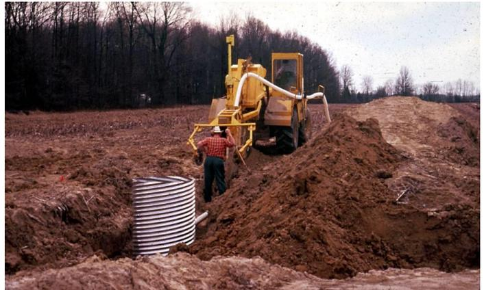
Photo 2. Lateral drain installation, exiting into culvert for measurement
