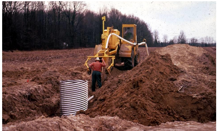
Photo 1. Lateral drain installation, exiting into culvert for measurement
