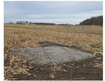
The blind inlet shown above was constructed with about 15 tons of steel slag which removed over 45% of the 3-yr DP load, plus >70% of glyphosate and dicamba. Note that blind inlets constructed with the traditional limestone material will not remove DP due to low calcium solubility.
