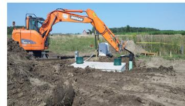
The subsurface tile drain filter above was designed to remove 40% of the 10-yr DP load, using only 2.5 tons of an iron-coated activated alumina material, a manufactured PSM. This material will be regenerated in-place after 10 years, through a [P-stripping technique](#) developed by USDA.
