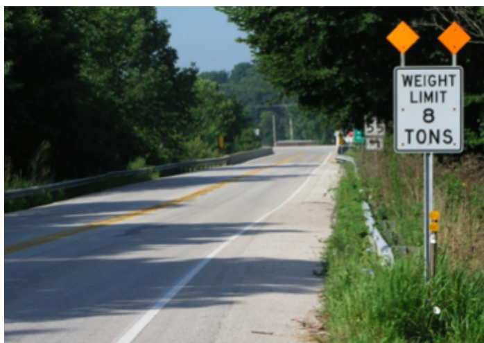
Figure 2. Bridges with Load Restrictions Must Have a Sign Posting the Allowable Load Limit
