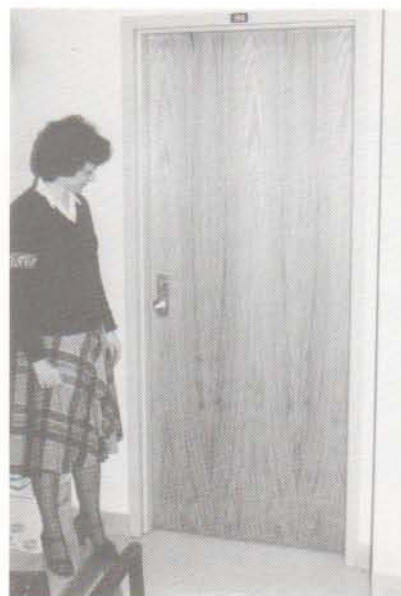
Figure 20. The four darker lines running from top to bottom of the door are mineral stain in red oak veneer.
