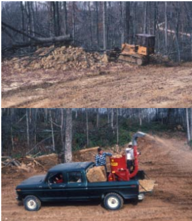
Log yards are often next to public roads or other high use areas. Cleaning up a log yard by grading ruts and seeding with native grasses and forbs improves its appearance and its value for wildlife habitat.
