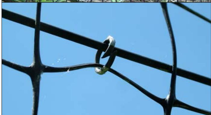
**Figure 10.** Use a hog-ring plier to attach the mesh to the monoline.
