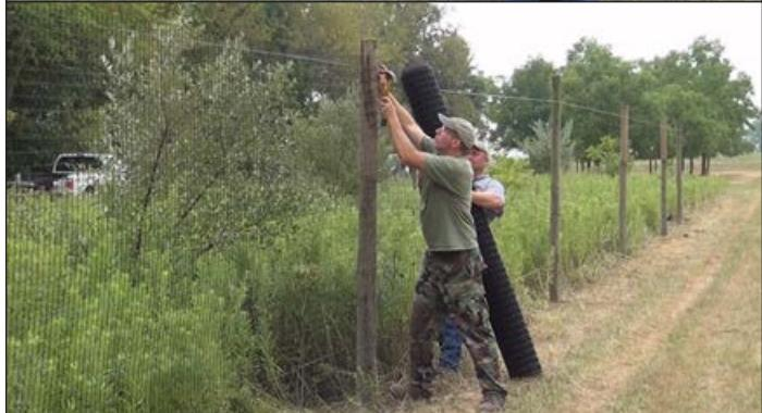
**Figure 9.** Position and nail the plastic mesh to the posts, being sure one square or about 2 inches of mesh are above the top monoline and 4 or 6 inches overlap the ground.
