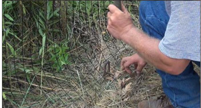
**Figure 11.** Stake the bottom of the fence once or twice between posts to reduce the pulling effects of the wind and to prevent deer from crawling under the fence.
