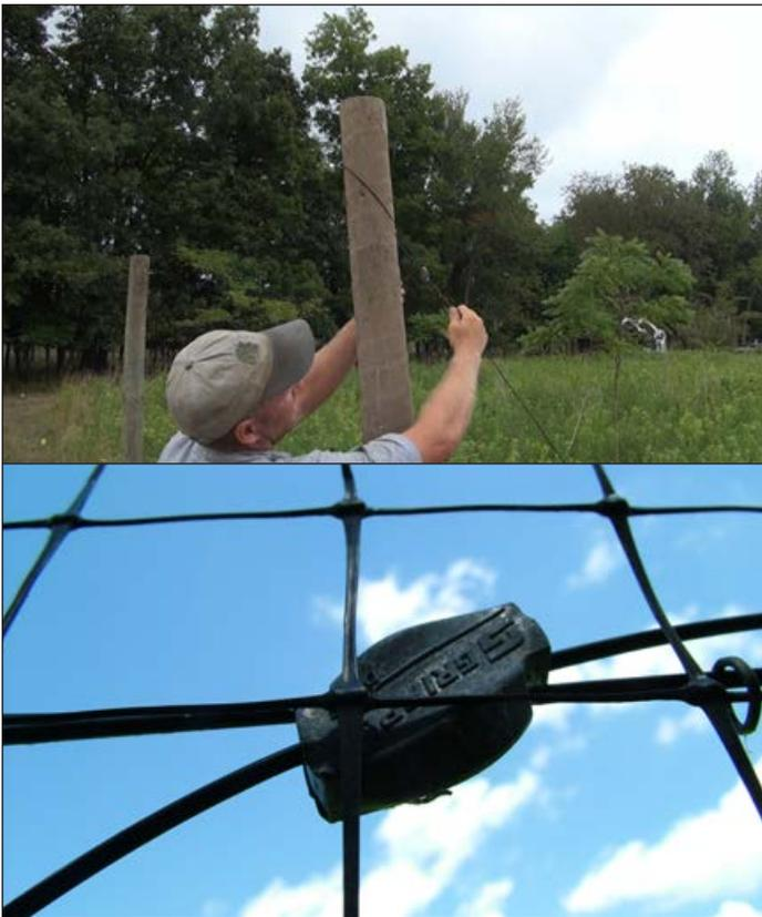
**Figure 6.** Secure the top monoline through a fence staple and attach a gripple.
