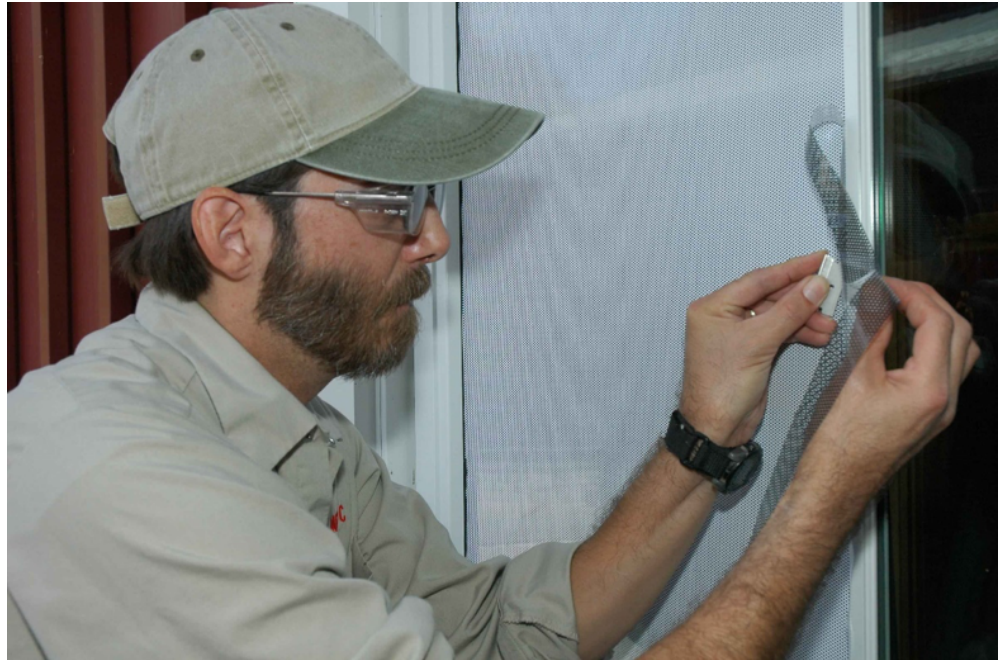
Figure 3. Application of one-way perforated anti-bird-strike film to a window (Photo by Billings Brett, U.S. Fish and Wildlife Service)
