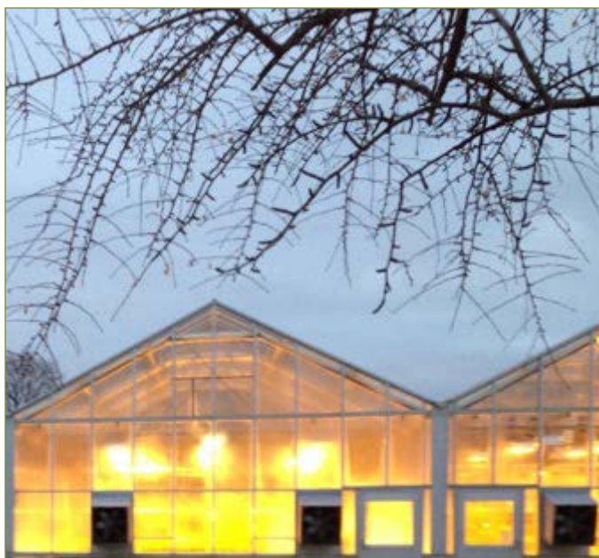
Figure 1. This greenhouse uses high-pressure sodium lamps to provide supplemental lighting.
