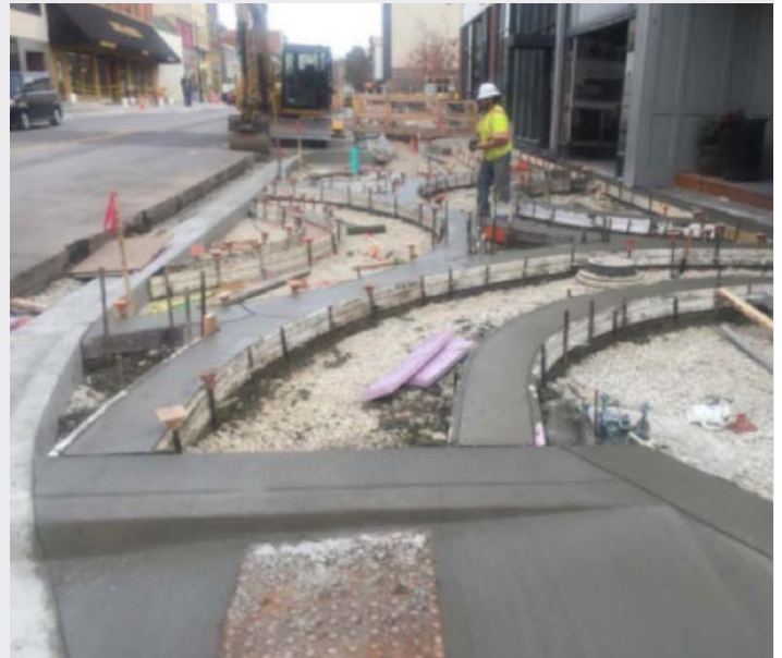
Figure 3: The image above shows expansion of the pedestrian environment through an intersection bulb-out. This area is now used for outdoor seating by a new restaurant that occupies the storefront to the right. Additional brick detail is featured within the concrete framework shown. The approach to the intersection has also been narrowed by this feature, slowing approaching traffic and allowing pedestrians to be clearly visible as they evaluate whether not it is safe to enter the crosswalk. Also note ADA compliant detectable truncated domes installed at the curb ramp. Photo courtesy of Bishop, Carson, Pohlar, 2017
