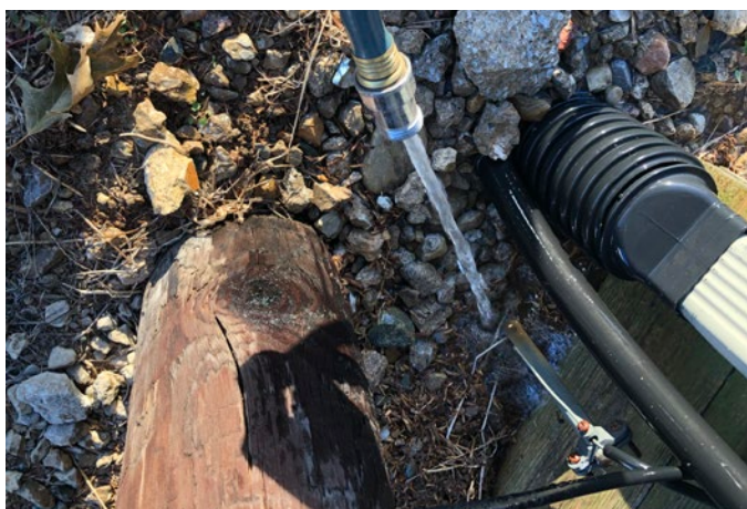
Figure 28. Adding water around the electric fence ground rods.
