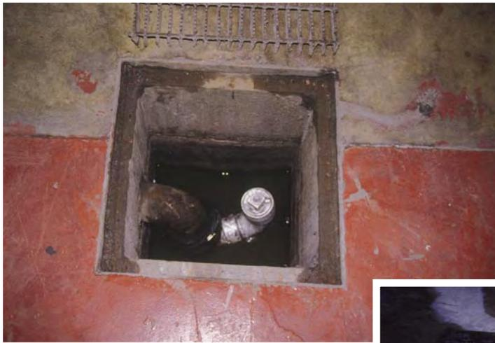
A PVC pipe is attached to the drainpipe (left) which is then extended upward with an elbow. The elbow is threaded to accommodate a screw cap.
