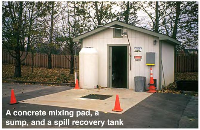
A concrete mixing pad, a sump, and a spill recovery tank
