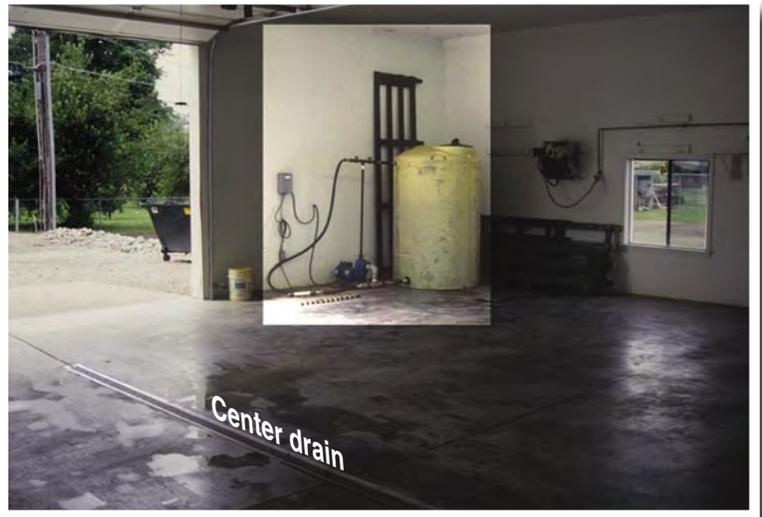
A lawn care company designed their floor to slope toward a center drain (above) which can be emptied into a holding tank in the back of the shop.
