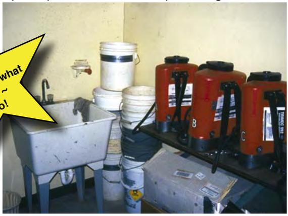
The pipe beneath the sink (right) is disconnected so that drainage is contained in a bucket. It is important to dispose of the bucket contents appropriately.
