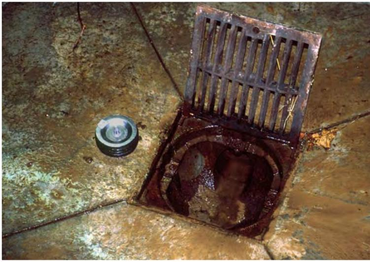
Expansion plug used to seal drain
