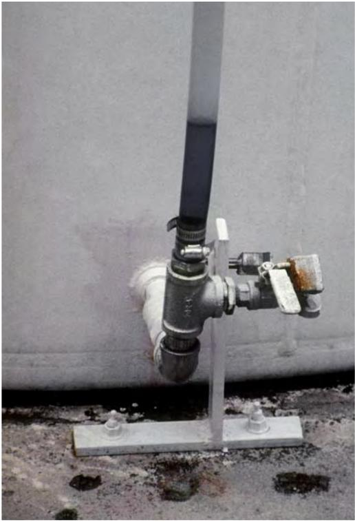
This photo shows a sight gauge locked on a tank.
