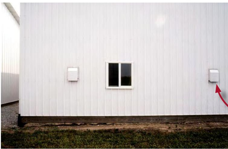
An air intake fan (above left and above) draws fresh air into the storage room. The clean air mixes with the storage room air and is drawn outside by another fan (above and left).
