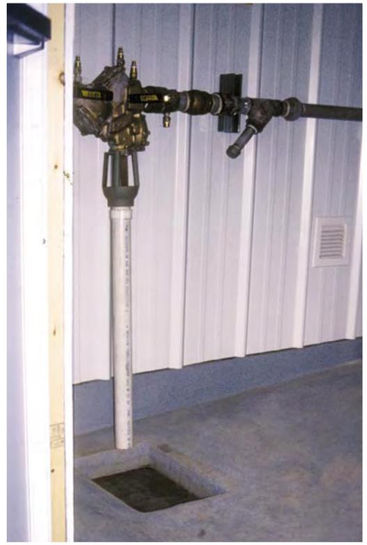
This is a backflow device to prevent siphoning of spray mixture into the well.
