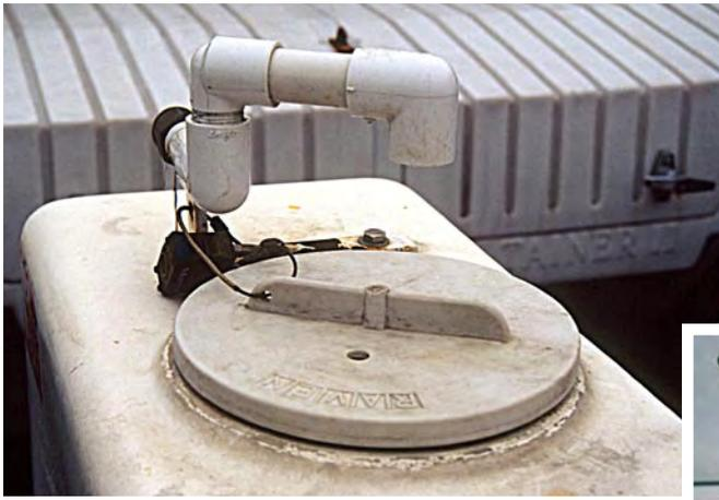
Tank lids are secured with a cable (left) and a padlock (below).
