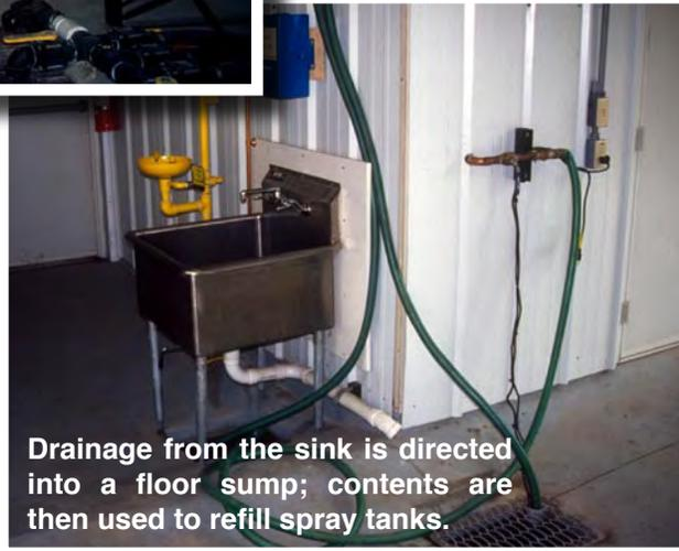
Drainage from the sink is directed into a floor sump; contents are then used to refill spray tanks.
