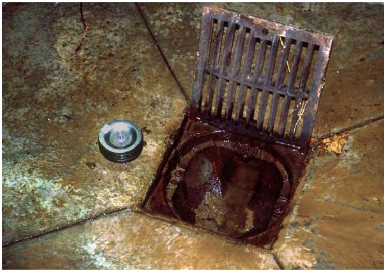
Plugs can be purchased to fit any opening. Turning the screw in the plug expands it to fill the opening.
