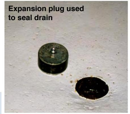
Plugs can be purchased to fit any opening. Turning the screw in the plug expands it to fill the opening.
