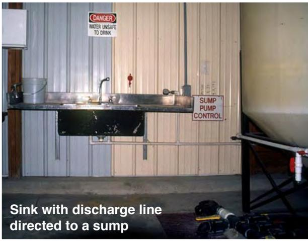
Sink with discharge line directed to a sump
