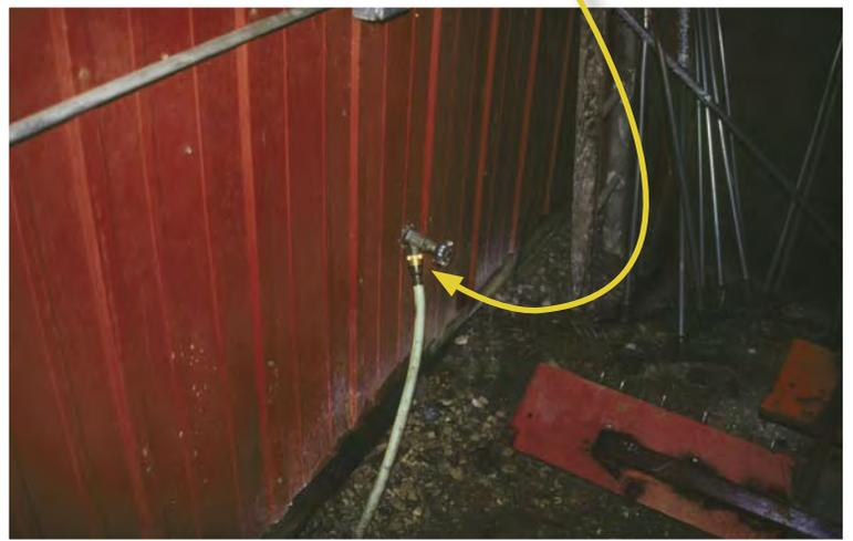
The backflow device installed in this water line is shown from two angles as the sprayer is being filled: at ceiling height (right) and from ground level (below).
