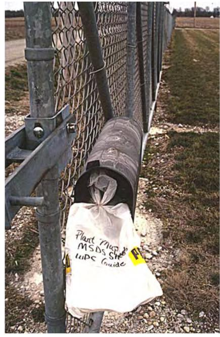
These are two examples of PVC pipes (with caps) that make excellent storage tubes for emergency information.
