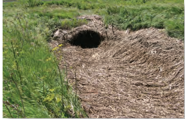
Debris-clogged ditches and drains can cause floods after heavy rains.
