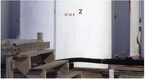
The clear hoses on these tanks gauge the level of fluid they contain. Only open the valve to these hoses when you want to check the level in the tank. If the hose fails when the valve is open, some or all of the tank's contents can be spilled.
