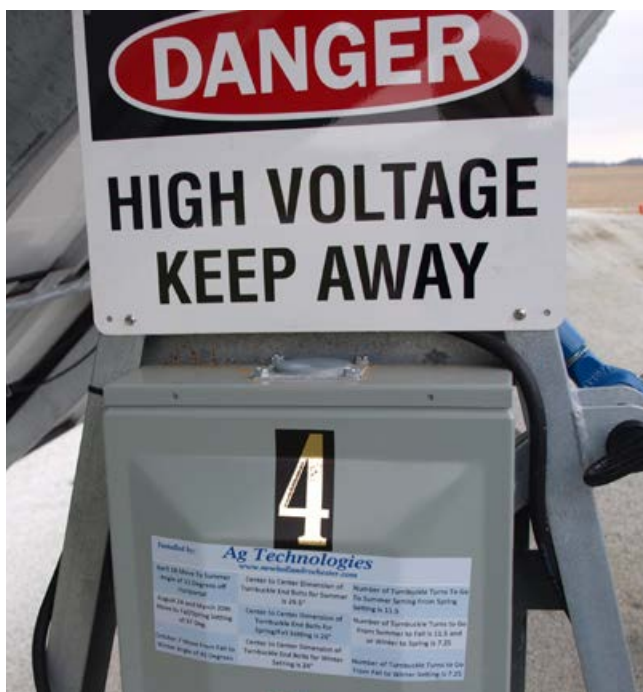
Toward the sun: This solar PV array includes instructions on how and when to adjust the system, increasing efficiency and reliability.
