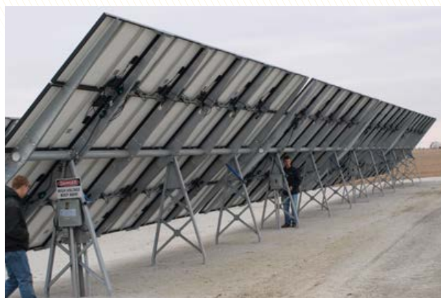
Big, small ... just right: Several factors influence the size and scale of a well-planned solar PV installation. Bigger may not be better. Determining the load demand is important.
