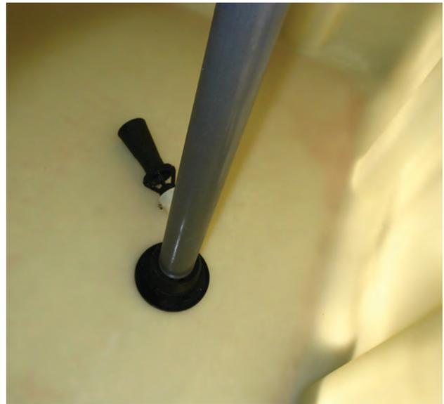
Ideally, agitation will be designed to constantly sweep the tank's bottom to prevent particle settling, either via use of bypass agitation or sparge bar systems.
