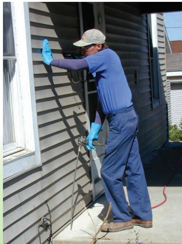
*Because his equipment is properly calibrated, this technician knows how long to apply insecticide in each injection hole to protect this home from termites.*
