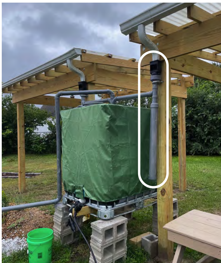
Figure 2: Rainwater harvesting system using an upcycled IBC tote covered with green waterproof nylon cover to minimize sunlight and algal growth. First flush diverter is circled in white to allow the first proportion of rooftop runoff to bypass the cistern.
